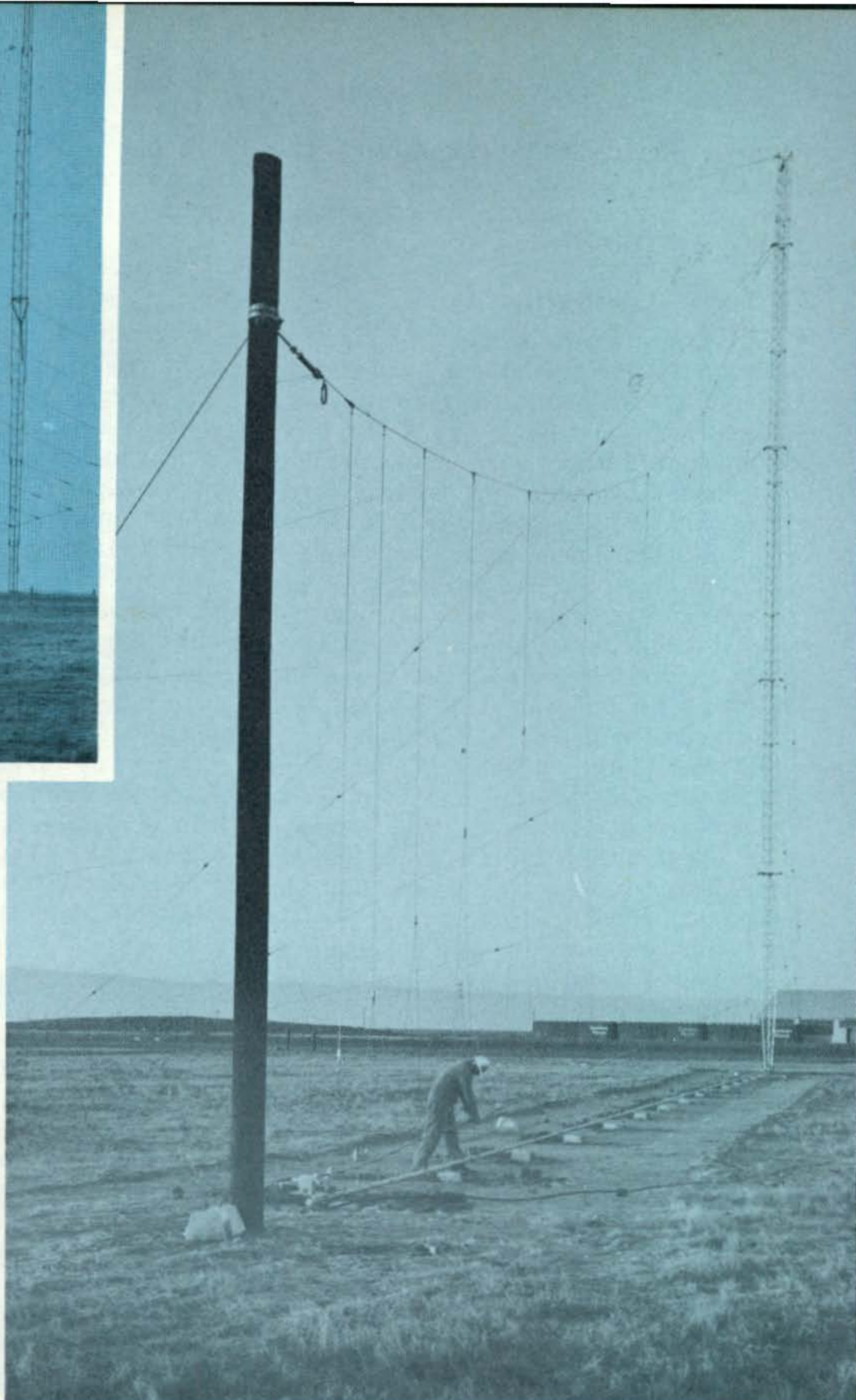
Photo 2 (bottom left)—A 20-60 mc LP dipole antenna, vertically polarized. Photo 3 (top left)—A Granger Transportable LP dipole for operation from 4 to 30 mc. Photo 4 (right)—A 3.5 to 32 mc vertical LP antenna.
